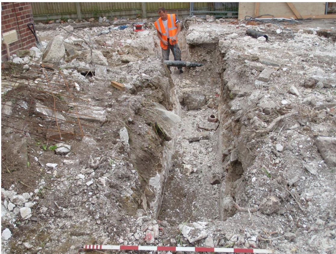
Plate 2. View of foundation trenches (looking NE)
