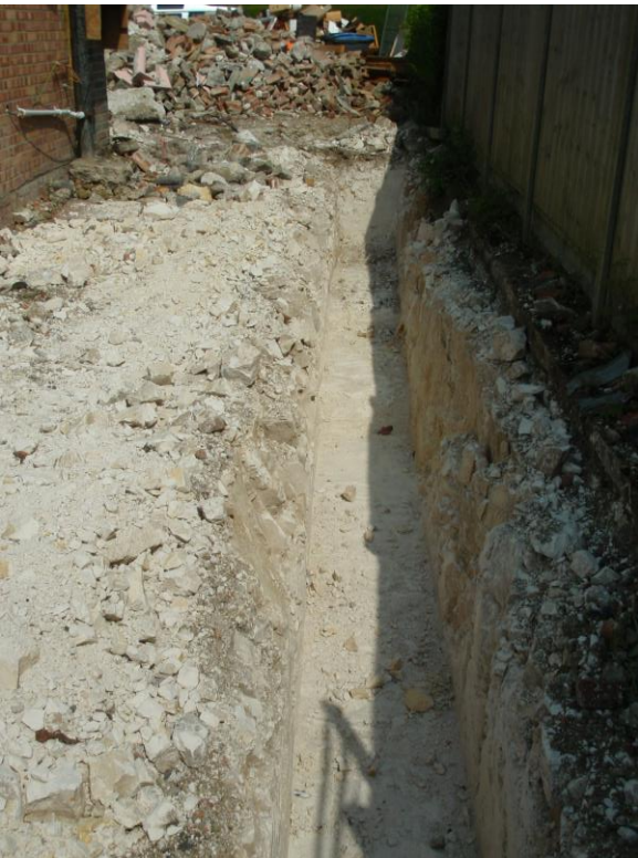
Plate 6. Foundation trench (looking NW)
