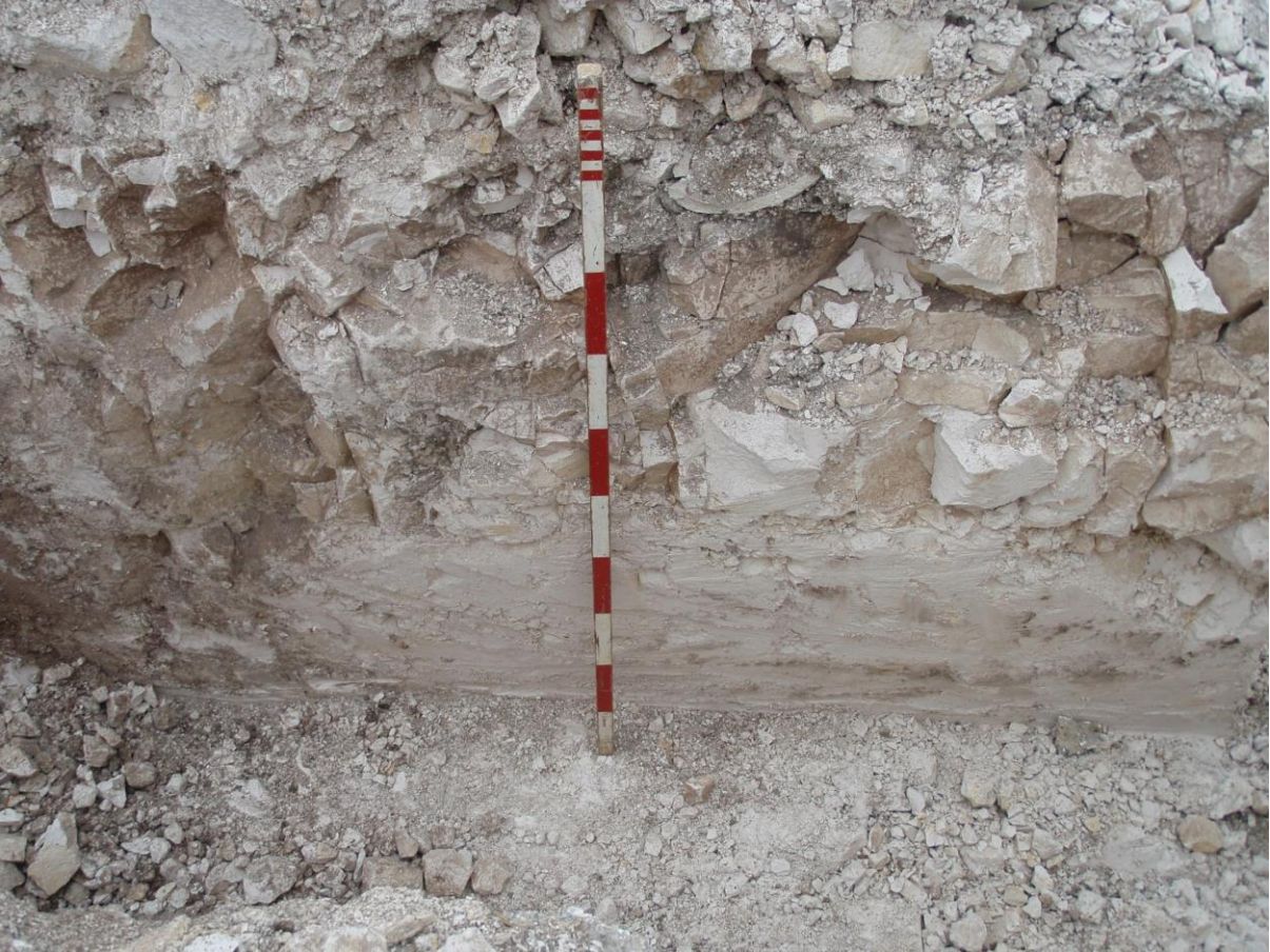
Plate 5. Foundation trench (section)
