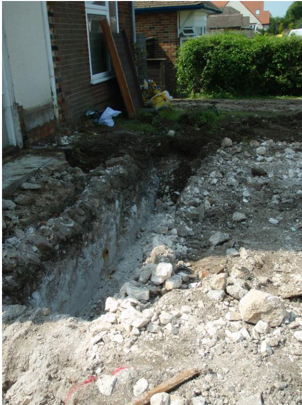
Plate 1. View of the foundation trenches (looking SW)
